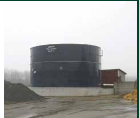
Right: Feeding a digester with thickened flush manure on a 900 cow sand bedded dairy in Western Washington.
